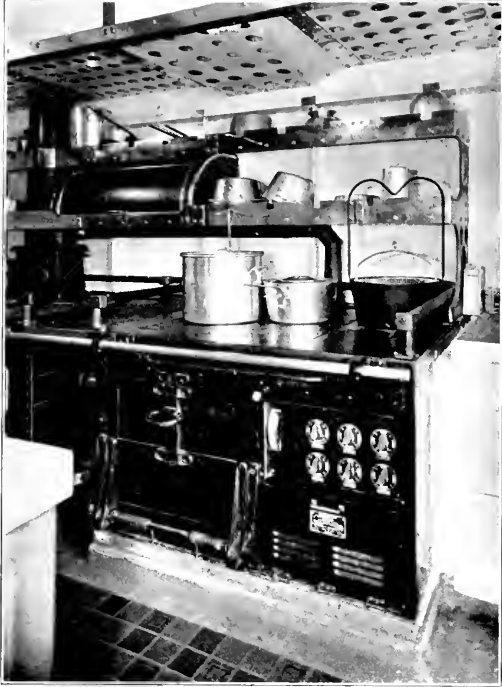
The galley is equipped with modern electric cooking apparatus specially designed for rough service at sea. Above is the Edison General Electric Appliance Co. range.
